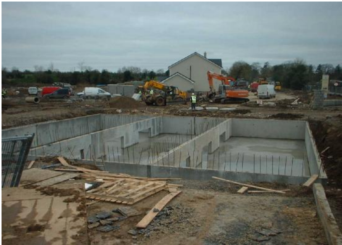
Typical Attenuation Tank in progress
