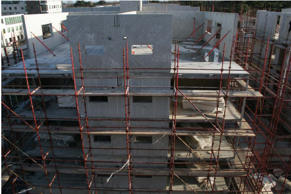
Building constructed with precast Walls & Floors
