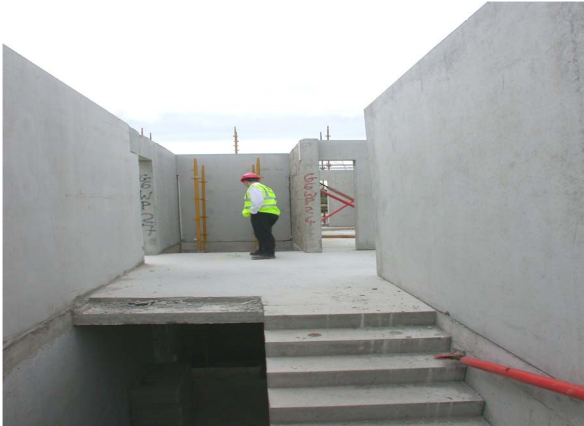
Precast Walls, Floors & Stairs
