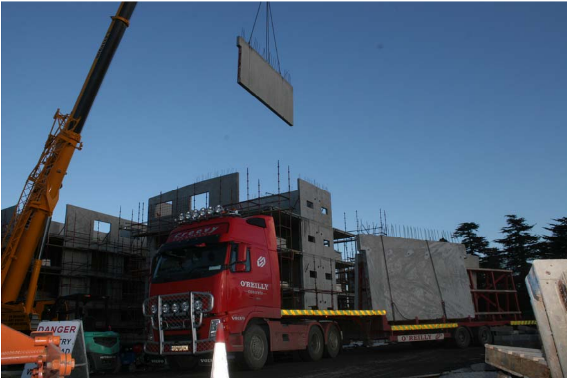
Walls unloaded from Trailers
