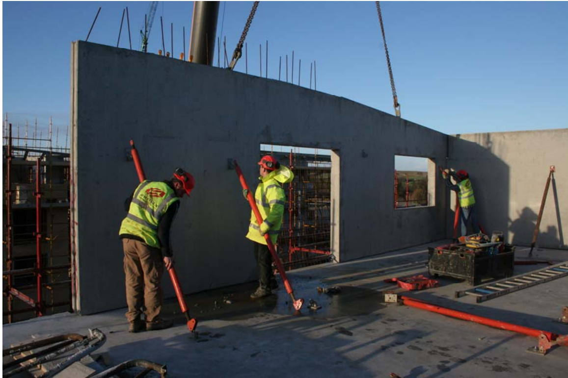
Walls propped and plumbed with Push-Pull props
