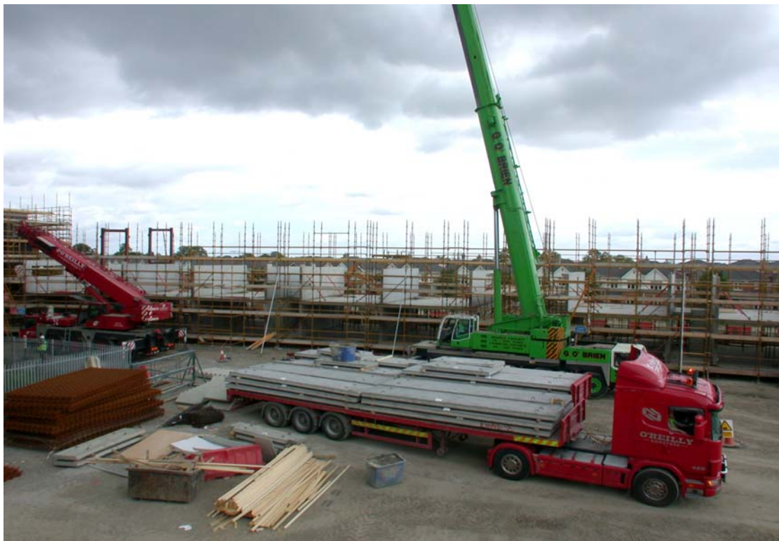
Prestressed Floors fitted on Precast walls
