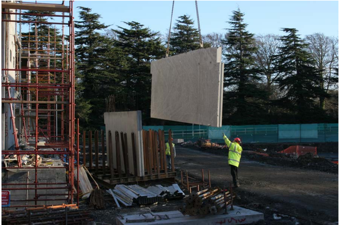
Walls stored on site in Wall Racks
