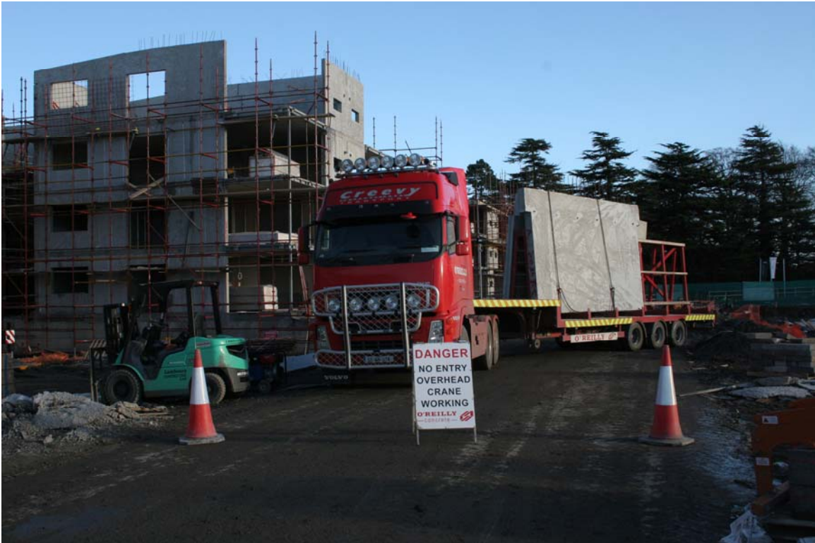
Walls Delivered to site on A-Frames
