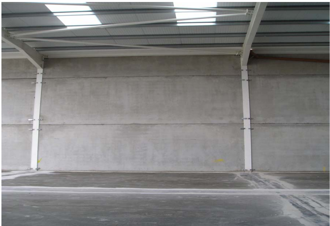
Battery Mould Walls used in warehouse
