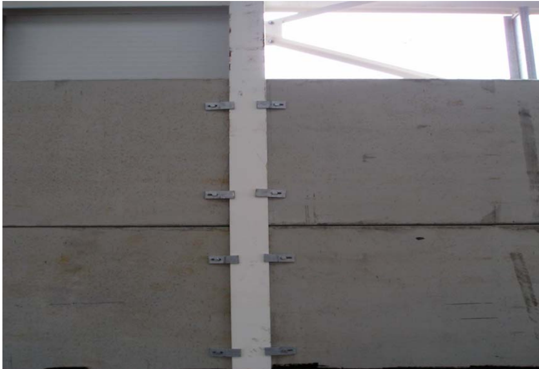
Walls clamped with Galvanised Plates
