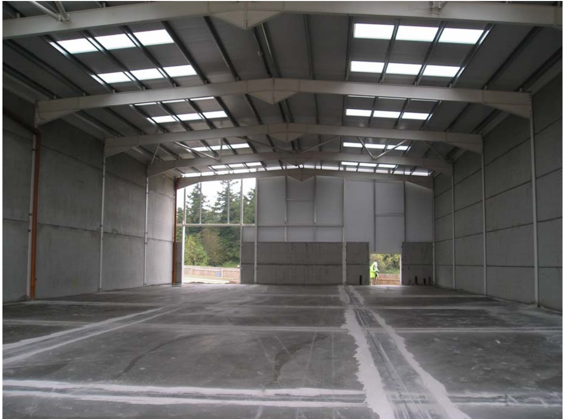
Battery Mould Walls used as Partition Wall
