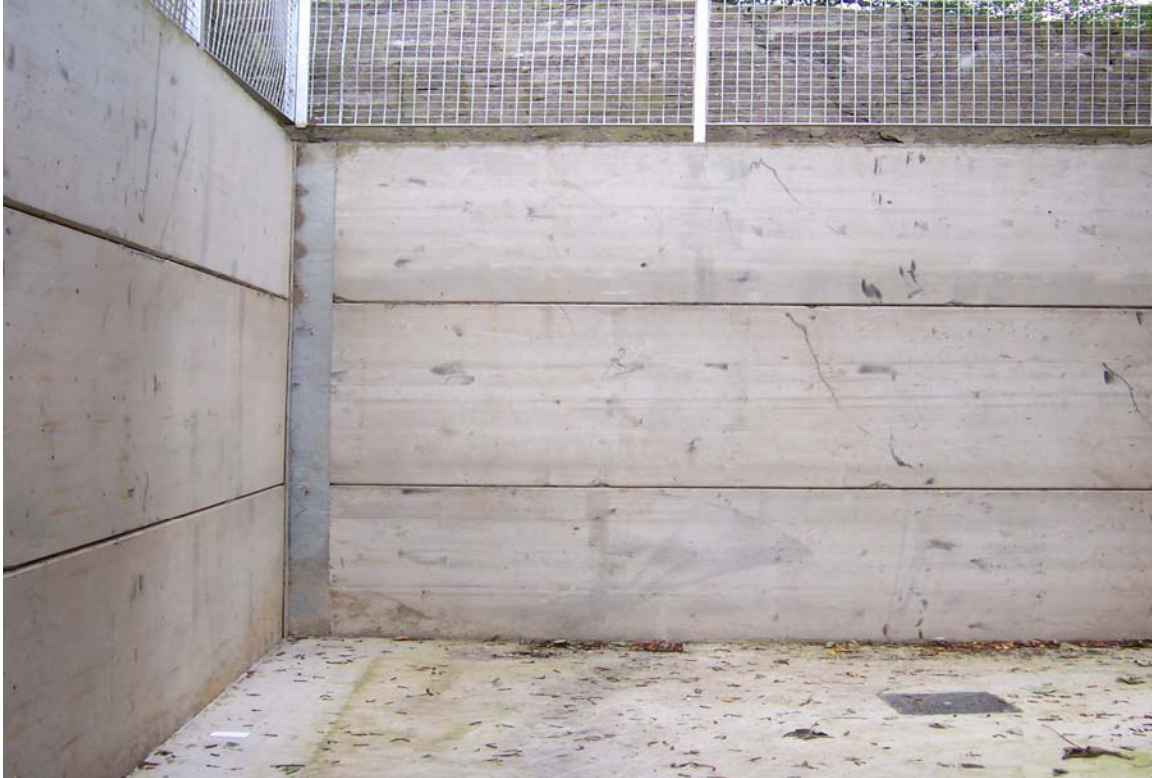
Retaining Clay Bank
