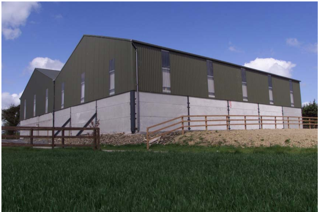
External Walls in Warehouse
