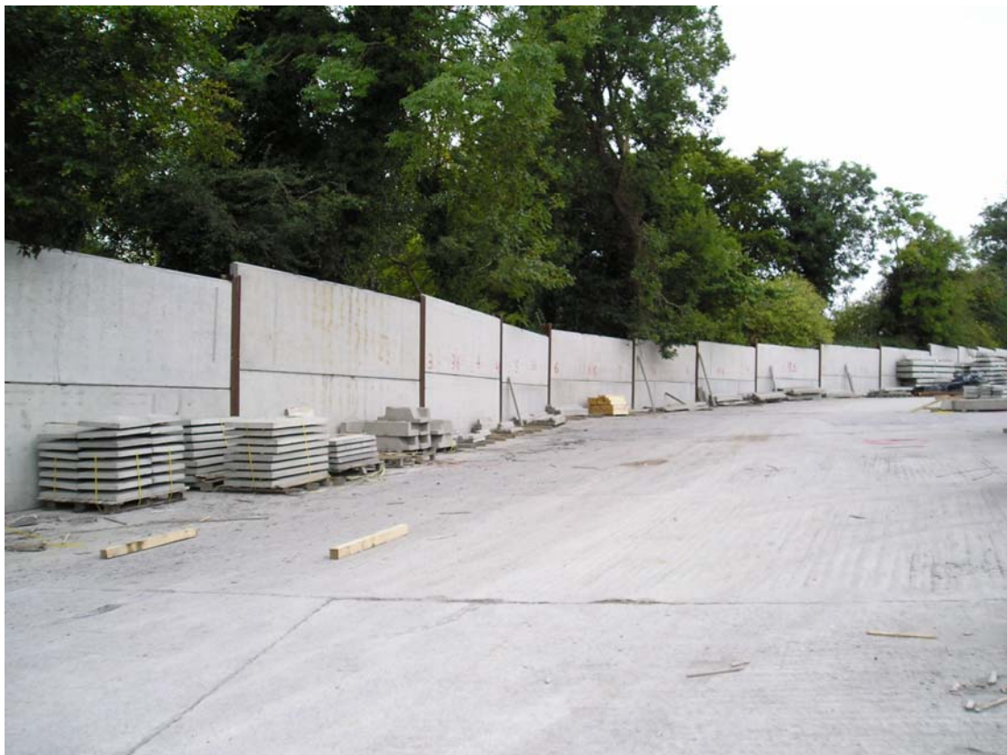
Stepped Wall on sloped ground
