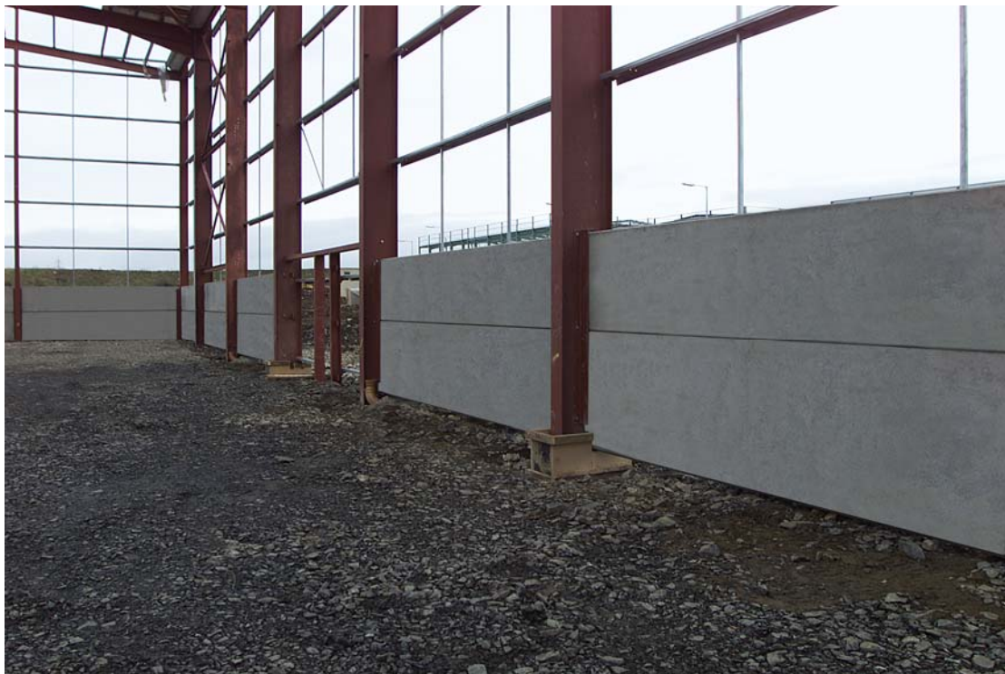
External wall in Warehouse
