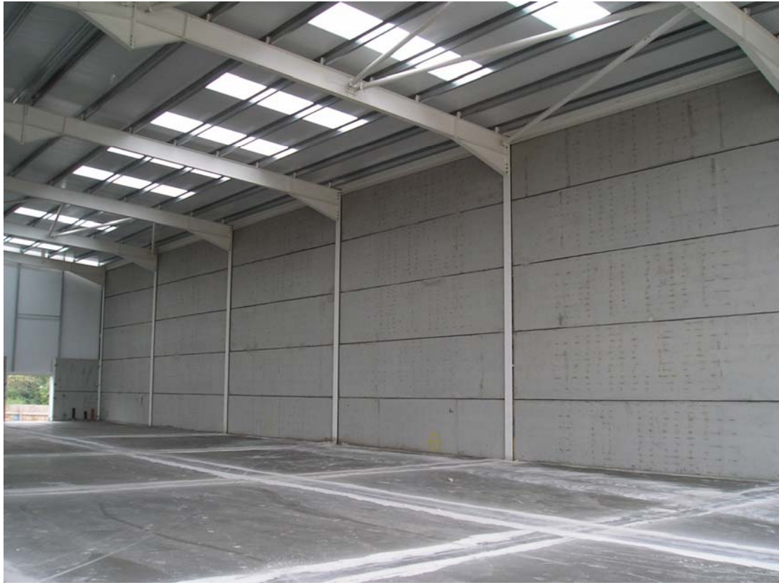
Dividing Wall in Warehouse
