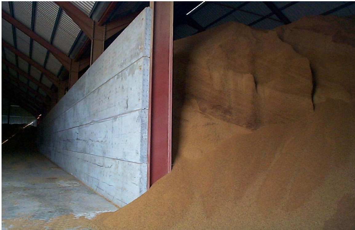
Retaining Wall in shed
