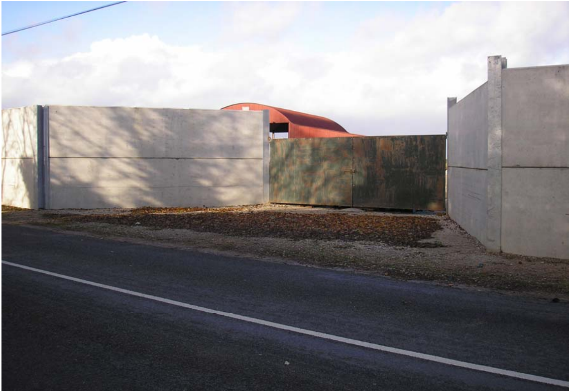
Entrance to Yard
