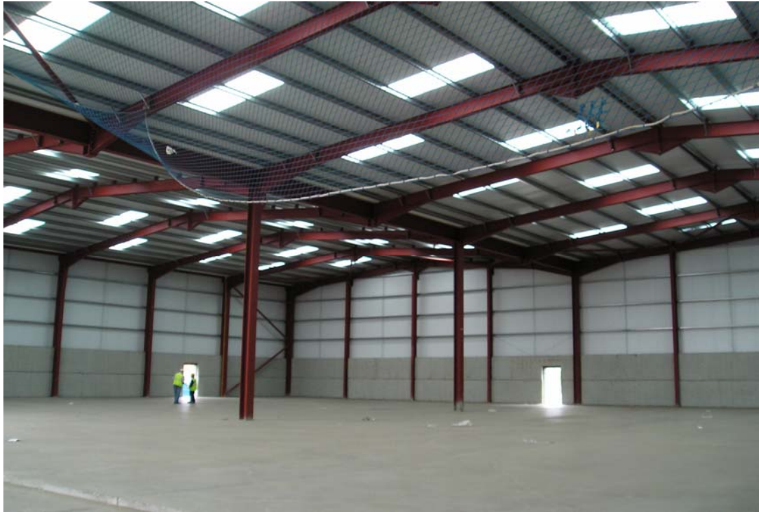
External Walls in Industrial Unit
