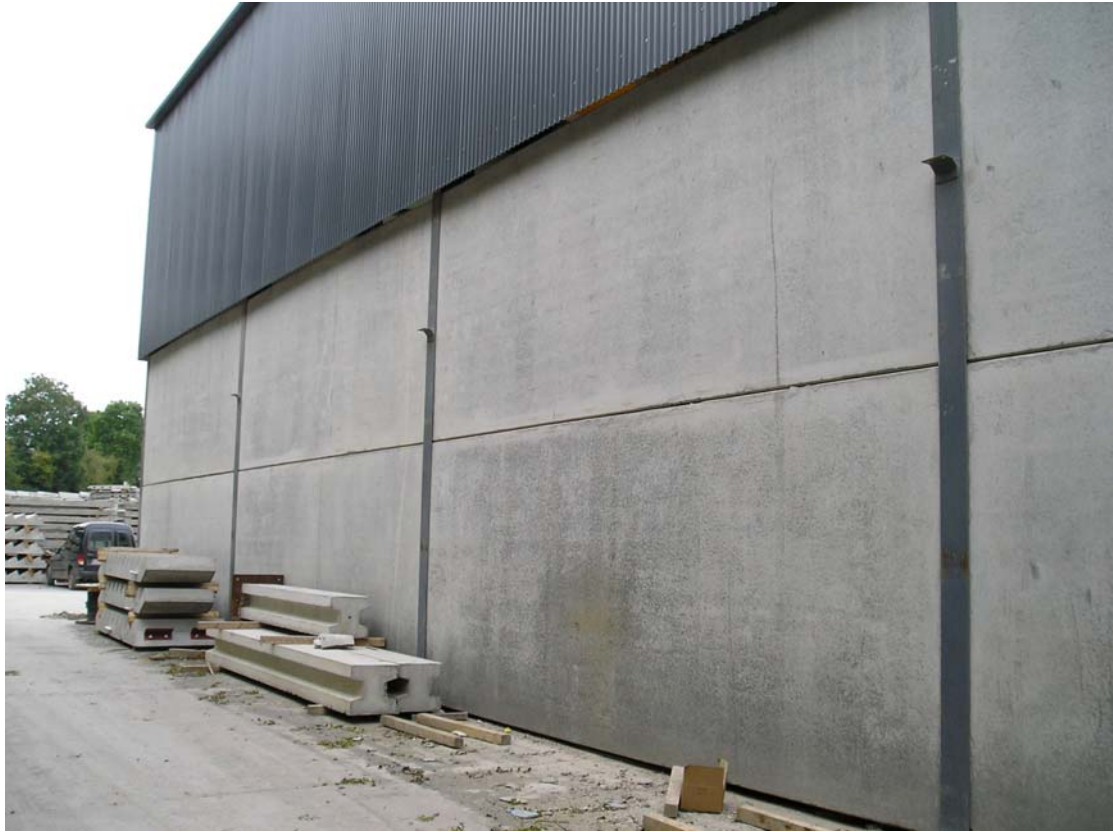
2.4 Meter Walls used in Shed
